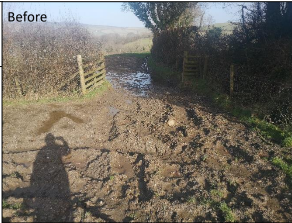
Culvert / Crossing point
