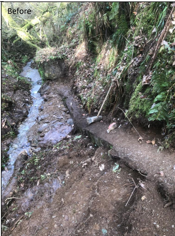
Ram Pump Repairs
