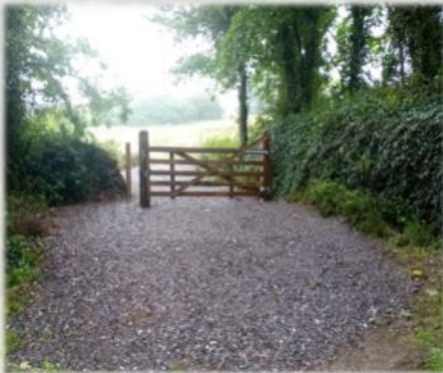
Access improvement work at Hillsborough southern entrance
